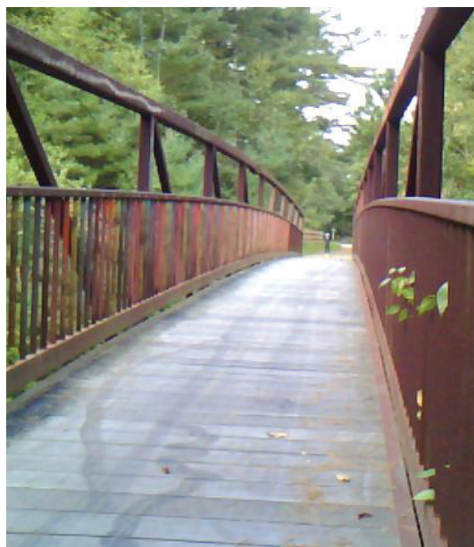
Moosup Valley Pedestrian Bridge
